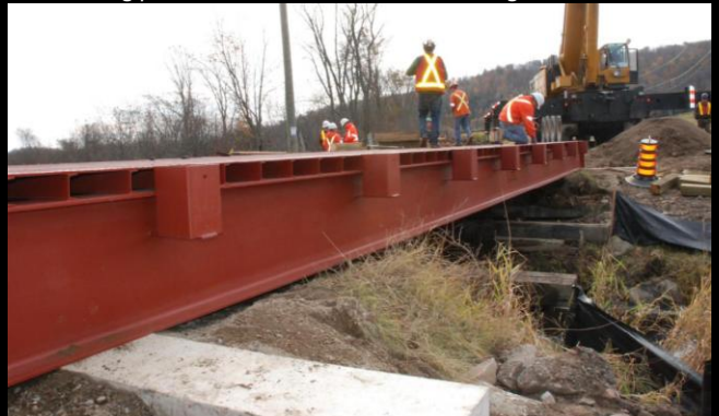
Photo 8: Downstream Face of new 18.3m span Lessard Modular Bridge.
